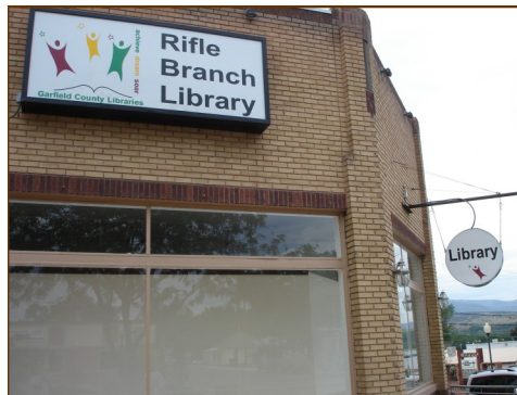
Rifle's temporary facility at 139 West 3rd Street.
