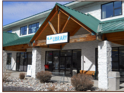
The temporary New Castle Branch Library.
