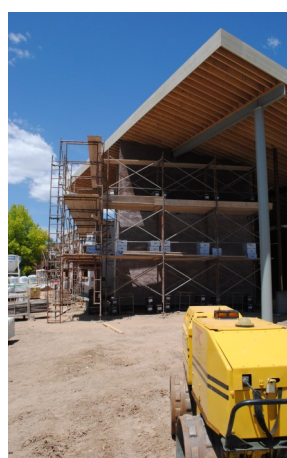
The new Silt Branch Library is taking shape quickly.
